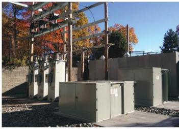
3-in-1 pad-mounted regulator with pad-mounted switchgear for bypassing to replace traditional overhead style regulators
