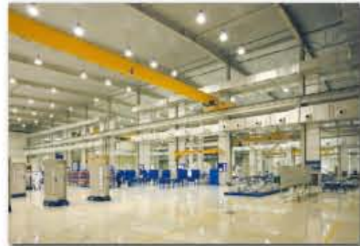
Final-assembly Workshop 1,000,000 Cleaning Grade, covers an area of 8,000m 2
